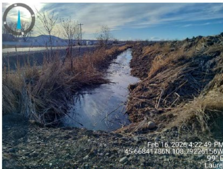
BED-AND-BANK-1, DREDGED SECTION
