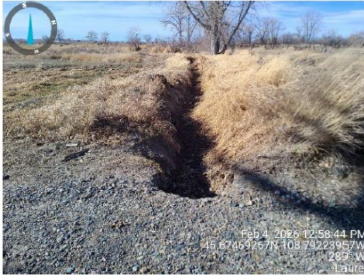
BED-AND-BANK-2, REPRESENTATIVE PHOTO
